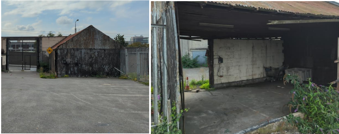
Plate 3: Derelict shed and concrete yard of the proposed Steeven's Lane substation site (left), and interior view of shed, with ivy ( Hedera helix ) and Buddleja observed on each side (right).
